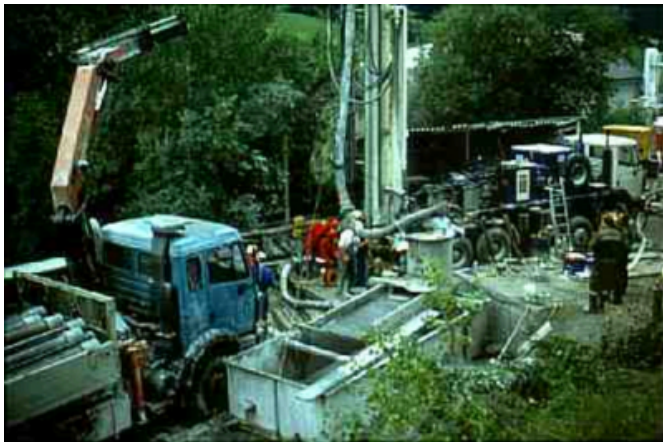
Image 6: Start of drill hole
